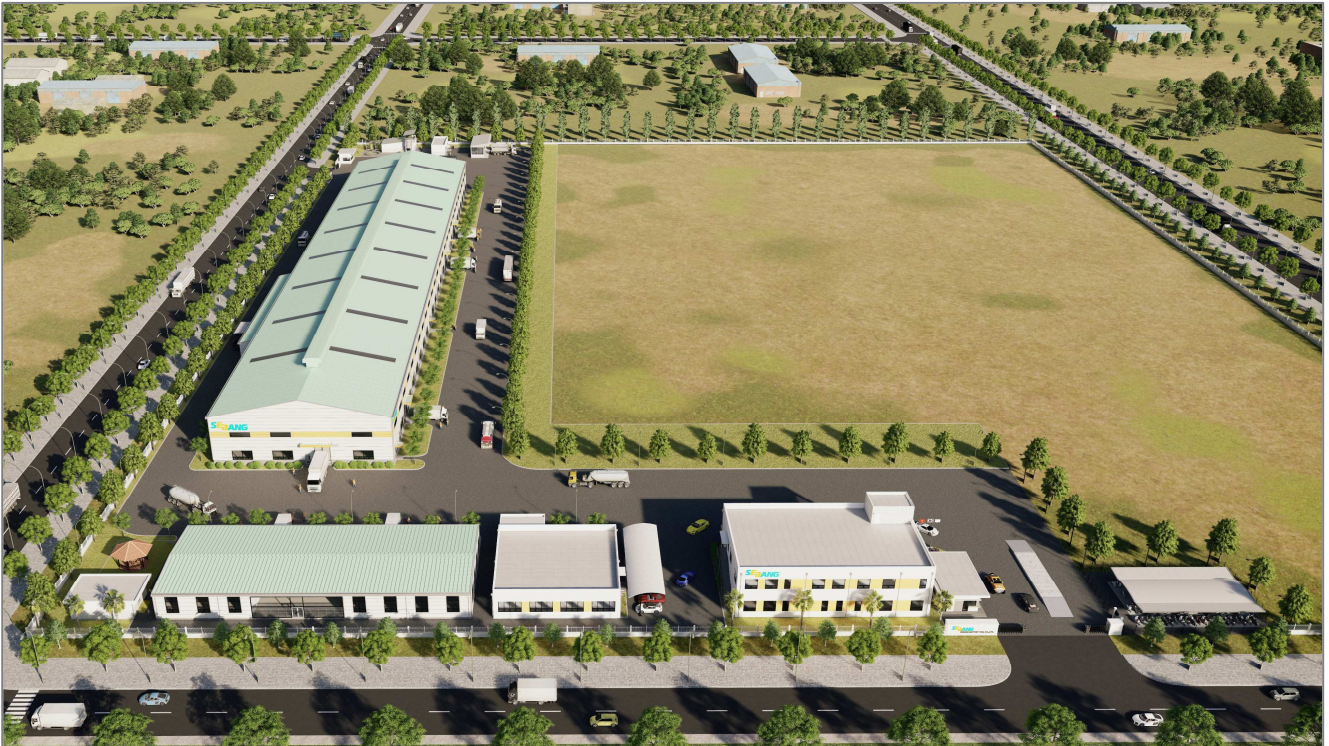
SEBANG BATTERY VINA FACTORY (2020, VIETNAM)
